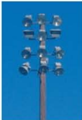
An example of luminaire mixes used for sports lighting in the 1980s. Note only two high-pressure sodium luminaires in a 12-luminaire bank.
