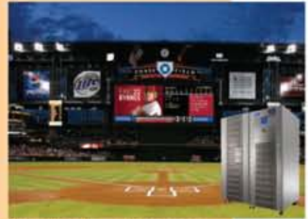
Chase Field, home of the Arizona Diamondbacks baseball team, recently updated its lighting and security lighting systems with central lighting inverters and 1,500-W metal halide fixtures.
