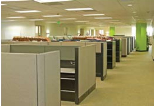
LiteGear Recessed T-Grid Ceiling with Indoor Fluorescent Fixtures (3) 32W Linear Fluorescent Lamps
